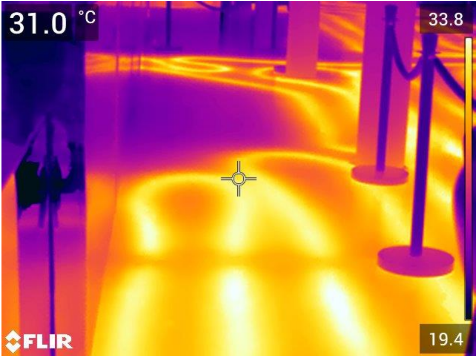
Hydronic Heating tracking via Thermal Camera
